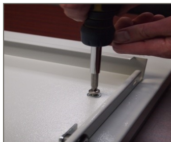
Figure 6: Attaching the sign bracket.
