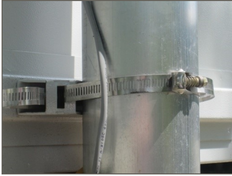
Figure 5: Sign Secured to a Pole with Banding Strap
