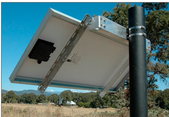
Figure 15: Solar panel mounting bracket
